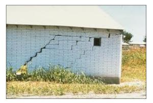
Fig. 1 Damage of the school due to a sliding plane not evidenced before
