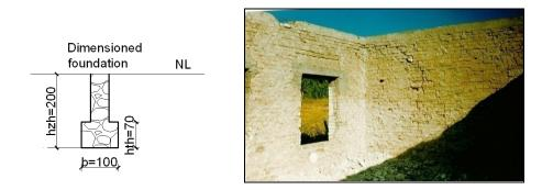
Fig 3 and 4 The dimensions of existing foundation (left) and wall cracks after 18 years of function (right).
